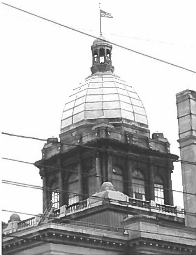
Figure 1 Tower and dome as seen today.
