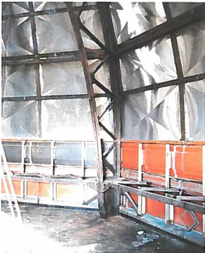
Figure 3 Structure at drum and lower dome.
