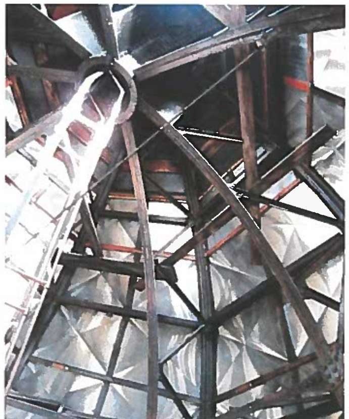
Figure 4 Compression ring at top of dome.
