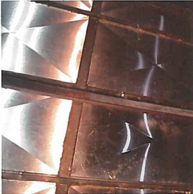
Copper clad metal armature originally supported the dome glazing.
