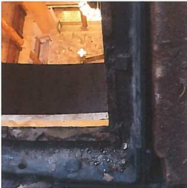
Metal clip securing wood trim to metal dome frame.
