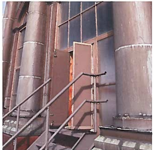
Access from clerestory to promenade deck.
