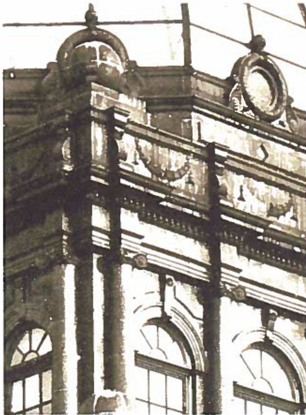
Original clerestory copper ornament circa 1915. Note missing swag above right window.
