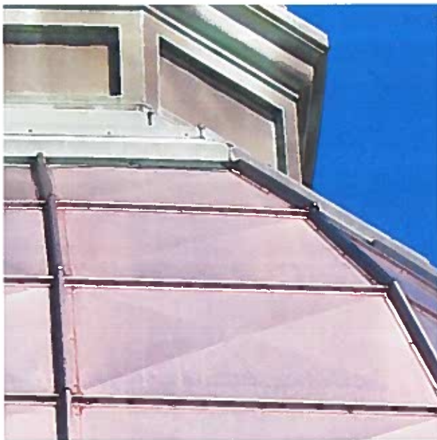
Stainless steel panels and ribs of the 1950s repairs.
