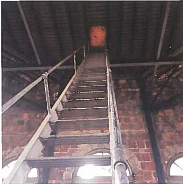
Ship ladder to dome. Note dome floor deck and joists.
