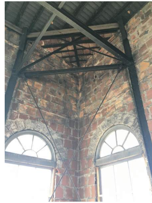
CLERESTORY SHOWING STRUCTURAL COLUMNS, STRUCTURAL CLAY TILE INFILL, AND WINDOWS
