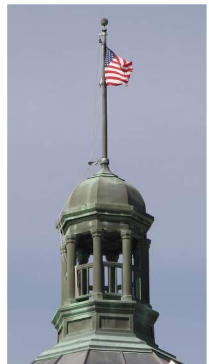
SIMPLIFIED LANTERN AND SKIRT. DOME IS FRAMED OVER ORIGINAL ROOF FRAMEWORK.
