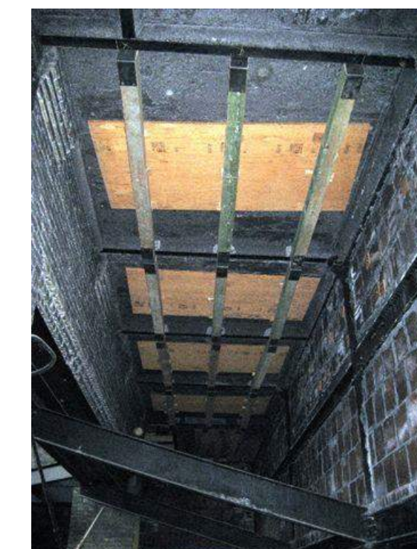
ATTIC VIEW OF REINFORCED CINDERCONCRETE PROMENADE DECK
