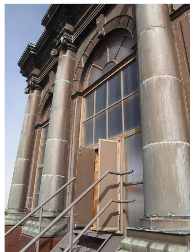
ALUMINUM ACCESS PANELS FROM CLERESTORY DEBRIS SCREEN LEVEL TO EXTERIOR PROMENADE DECK. WINDOWS ARE REPLACEMENTS
