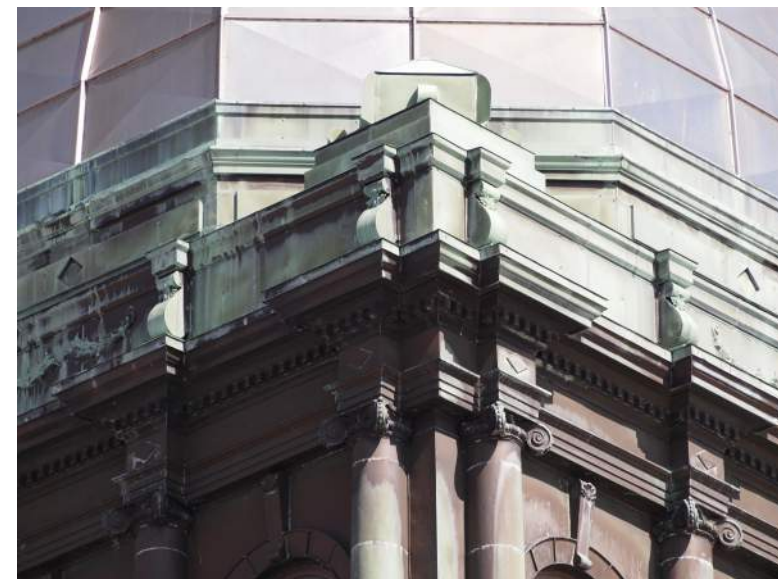
ORIGINAL ENTABLATURE, SIMPLIFIED REPLACEMENT BRACKETS AND CORNER ORNAMENT
