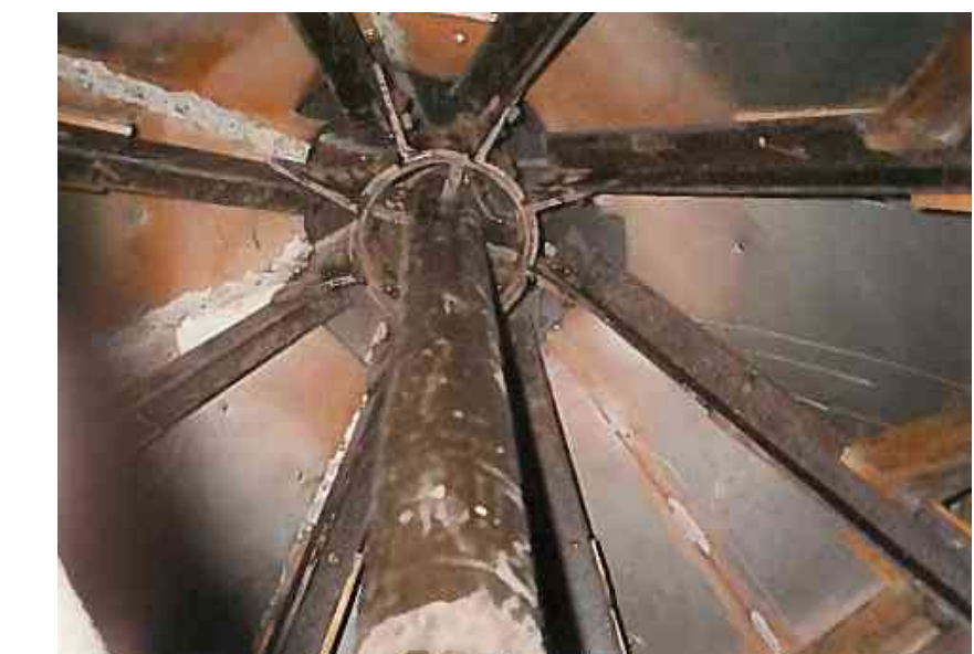
ORIGINAL LANTERN FRAMING WITH FLAGPOLE INSERTED AND WOOD FRAMING INSERTED TO CREATE EXISTING LANTERN DOME
