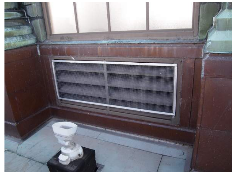
CENTER BAY BAROMETRIC RELIEF LOUVER, EACH ELEVATION. NOTE ARCHITECTURAL UPLIGHTS
