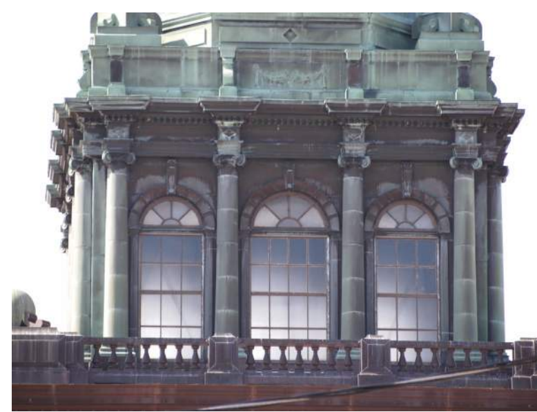
CURRENT CLADDING (ORIGINAL AND ALTERATIONS)
