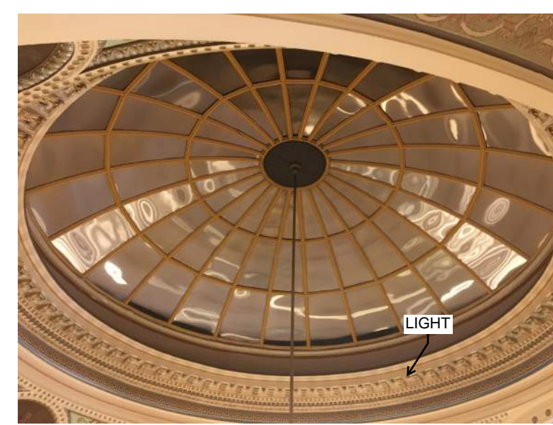
ATRIUM INTERIOR DOME FROM ATRIUM SHOWING UNDERSIDE OF CORNICE AND LIGHTS BETWEEN MODILLION BRACKETS
