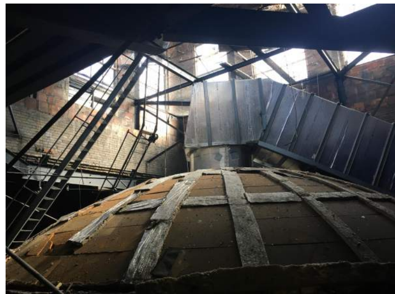
INTERIOR ATRIUM DOME (INSULATED) AND CURRENT RETURN AIR DUCT BELOW BASE OF CLERESTORY
