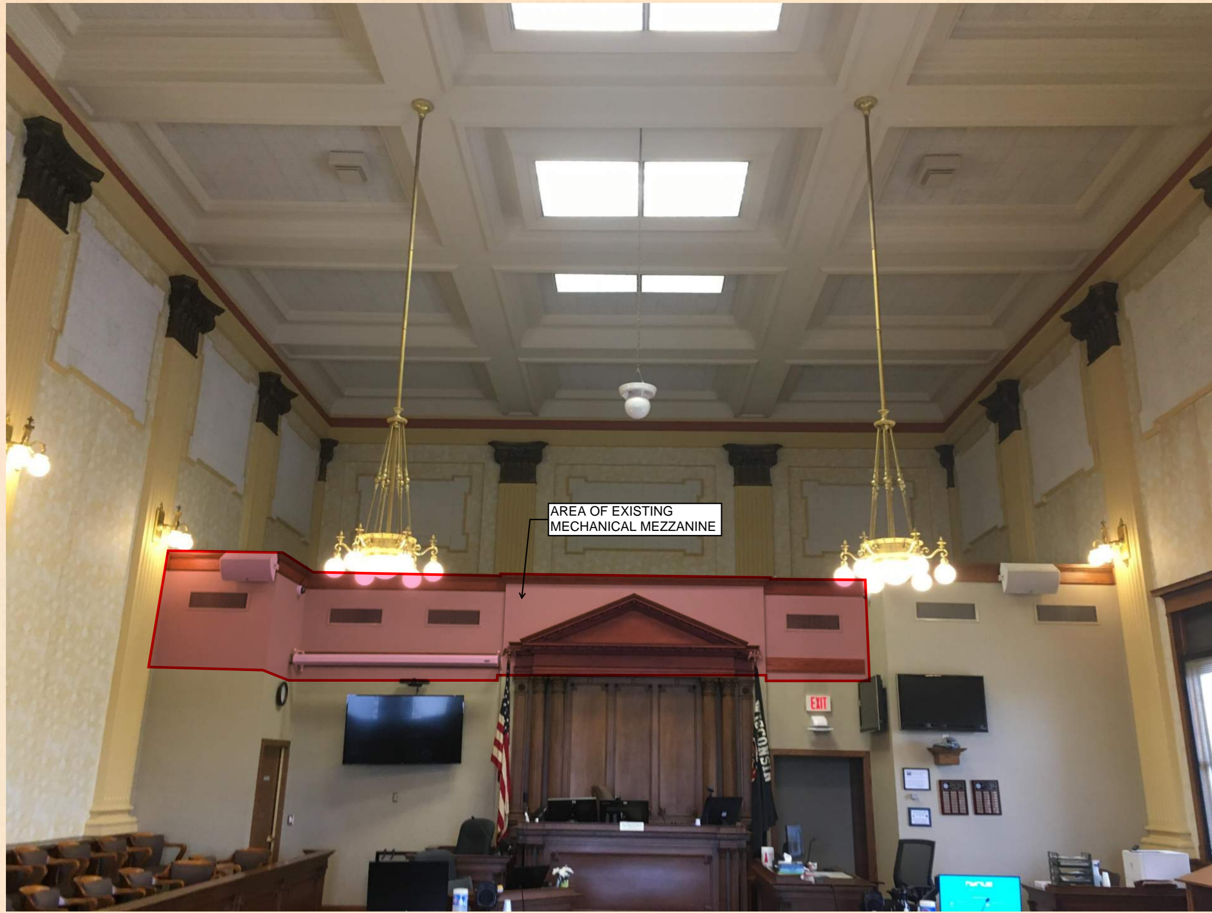
COURTROOM LOOKING EAST TOWARDS COURT OFFICES BUILT INTO COURTROOM
