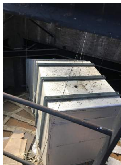
CHANDELIER SUPPORT CABLE THRU RETURN AIR DUCT
