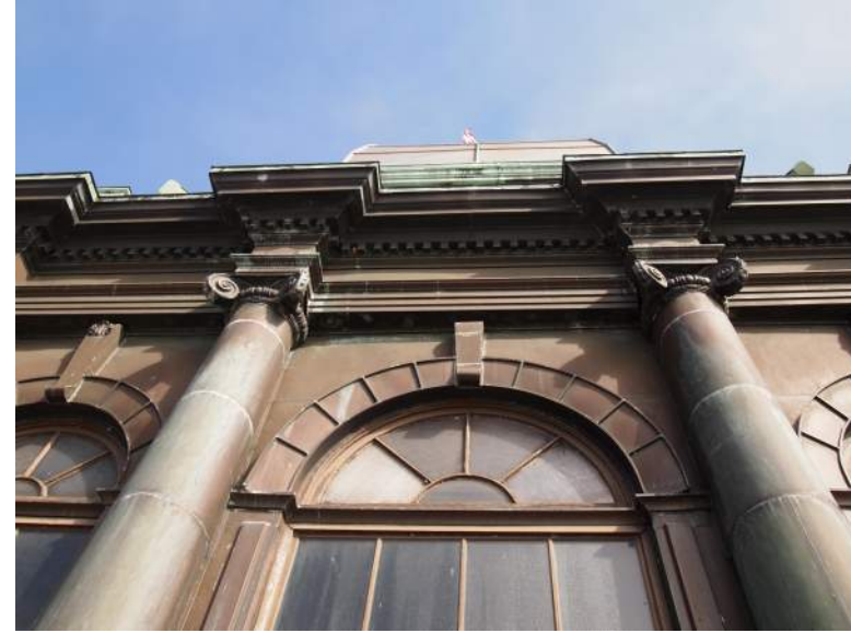
ORIGINAL WOOD SUNBURST WINDOW FRAME AND SASH, SIMPLIFIED WINDOW SURROUND ORNAMENT
