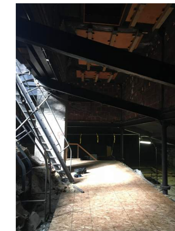
VIEW OF ATTIC AROUND ATRIUM DOME (TO LEFT)
