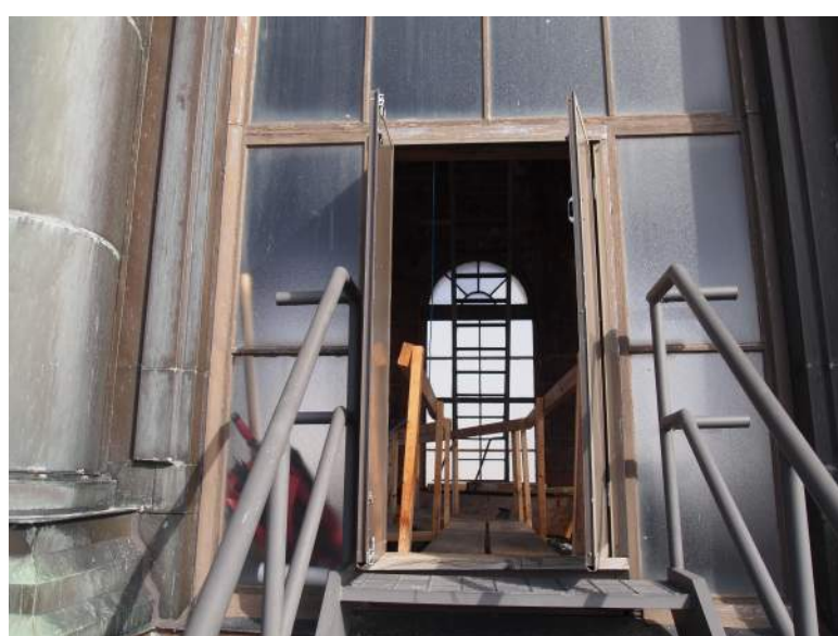
ALUMINUM ACCESS PANELS FROM CLERESTORY DEBRIS SCREEN LEVEL TO EXTERIOR PROMENADE DECK. WINDOWS ARE REPLACEMENTS
