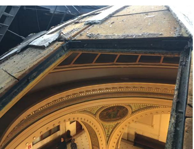
VIEW OF ATRIUM THRU REMOVED PANEL IN ATRIUM INTERIOR DOME
