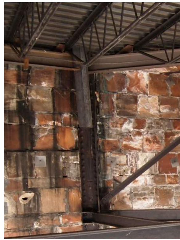
EXTENSIVE STRUCTURAL CLAY TILE WATER DAMAGE AND CORROSION OF TOP OF COLUMN/CONNECTION TO DOME TRUSS
