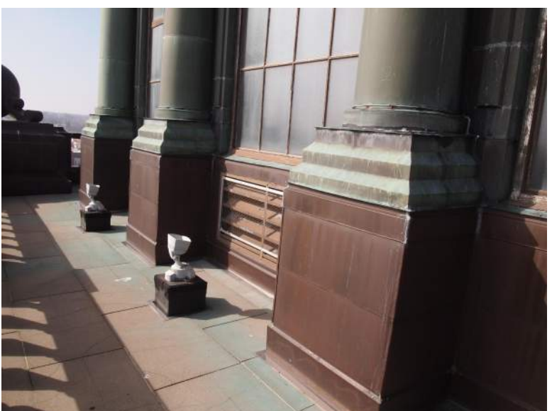
SIMPLIFIED COLUMN BASE REPLACEMENTS AND PLINTH CAPS. NOTE ARCHITECTURAL UPLIGHTS
