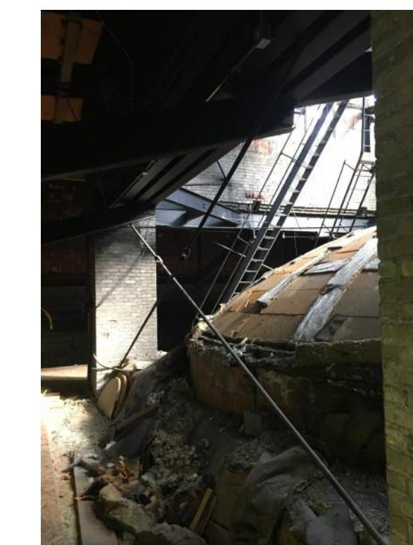
VIEW OF ATTIC AROUND ATRIUM DOME, NOTE STAIR TO DOME AND ABANDONED LADDER IN BACKGROUND
