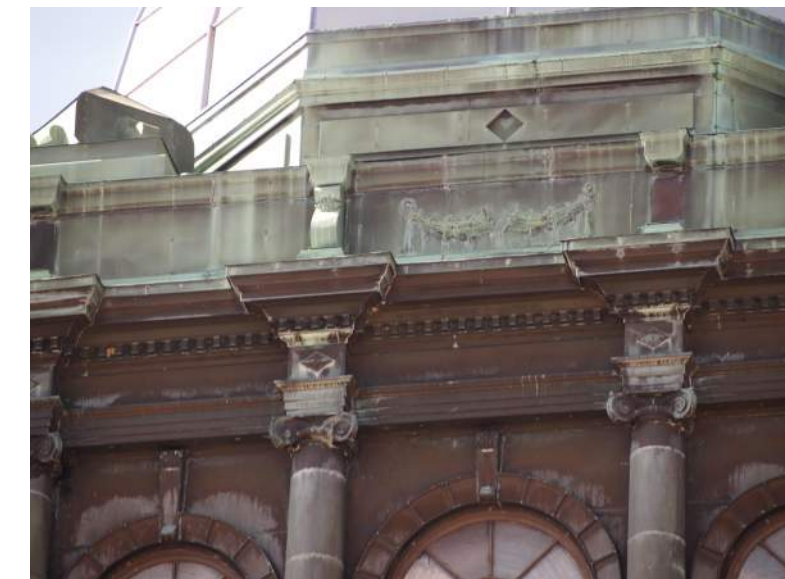
NOTE ORIGINAL STAMPED SWAG ORNAMENT ABOVE ENTABLATURE AND ON REPLACEMENT BRACKETS
