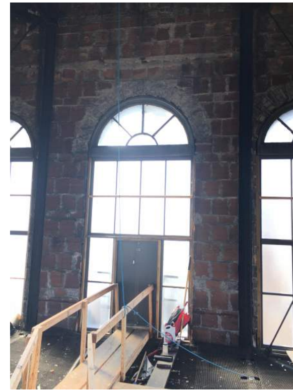
WEST ELEVATION PROMENADE ACCESS DOORS AND CATWALK OVER DEBRIS SCREEN
