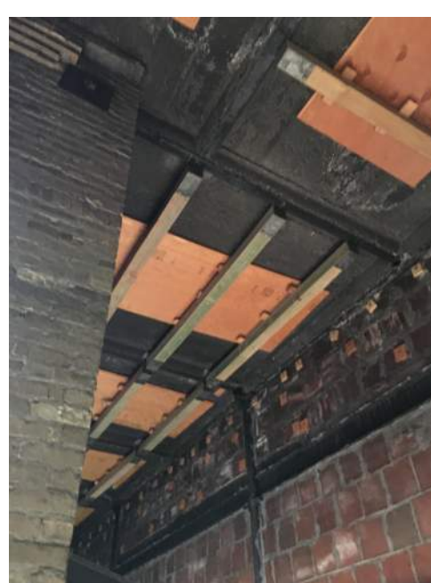
ATTIC VIEW OF REINFORCED CINDERCRETE PROMENADE DECK
